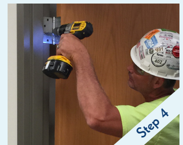
Doors installed on-site
